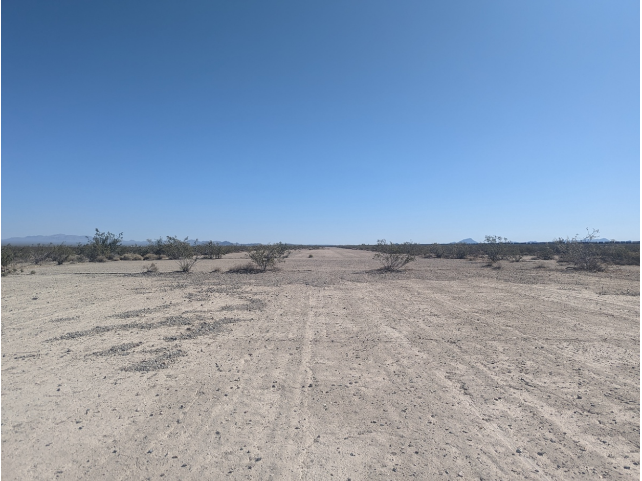
Figure 11: Remains of a taxiway
