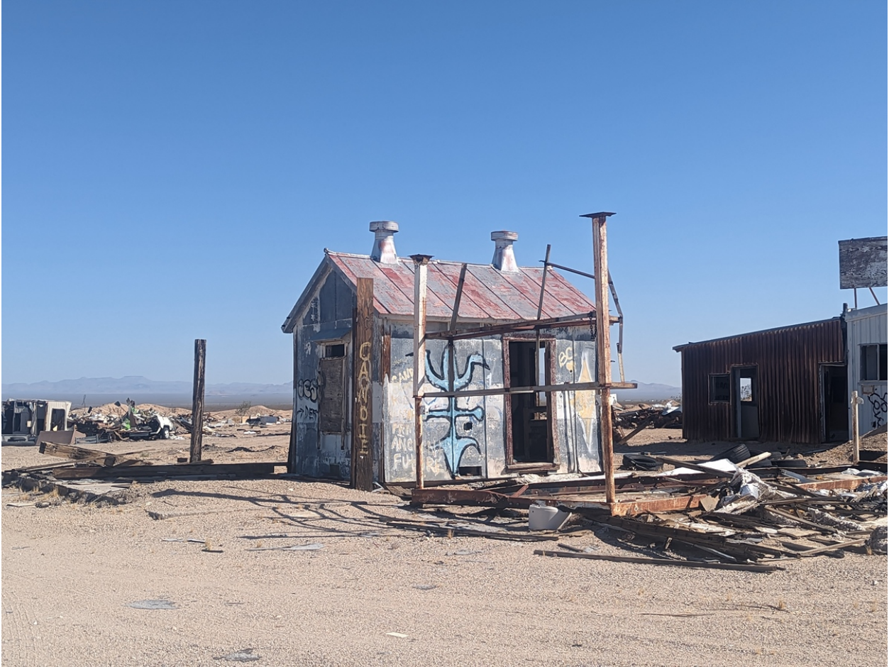
Figure 9: A sheet metal shed
