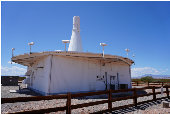
Figure 6: Rear of building
